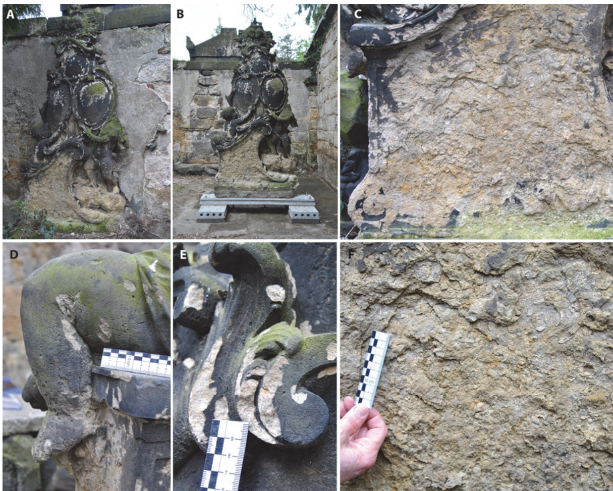
Fig. 1.2: Damage pattern of the baroque tombstone. A: Original place of the tombstone; B: Translocation of object before treatment; C: Relief, complete loss of original surface; D: Cracks; E: Missing part; F: Flaking
