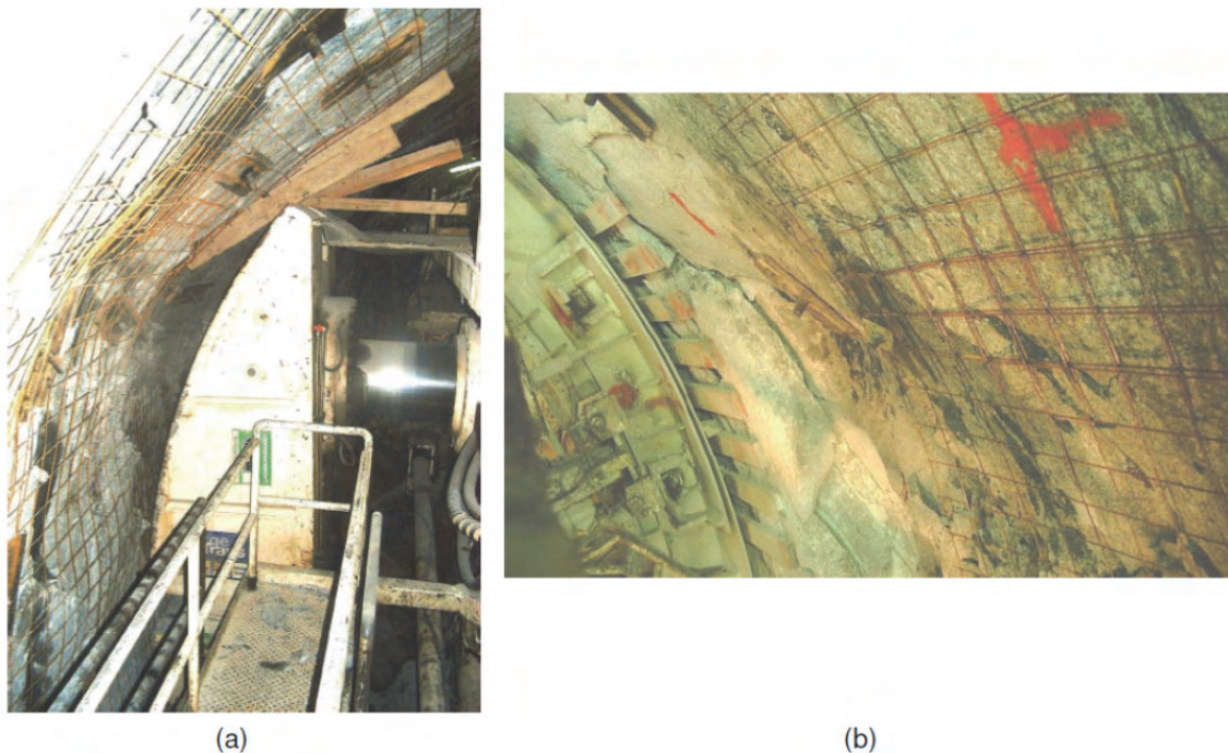
Fig. 3.1: Severe operational issues (gripper pads cannot be seated on the sidewall) associated with overbreak (notch) in the Lötschberg Base Tunnel (Loew et al., 2010).
