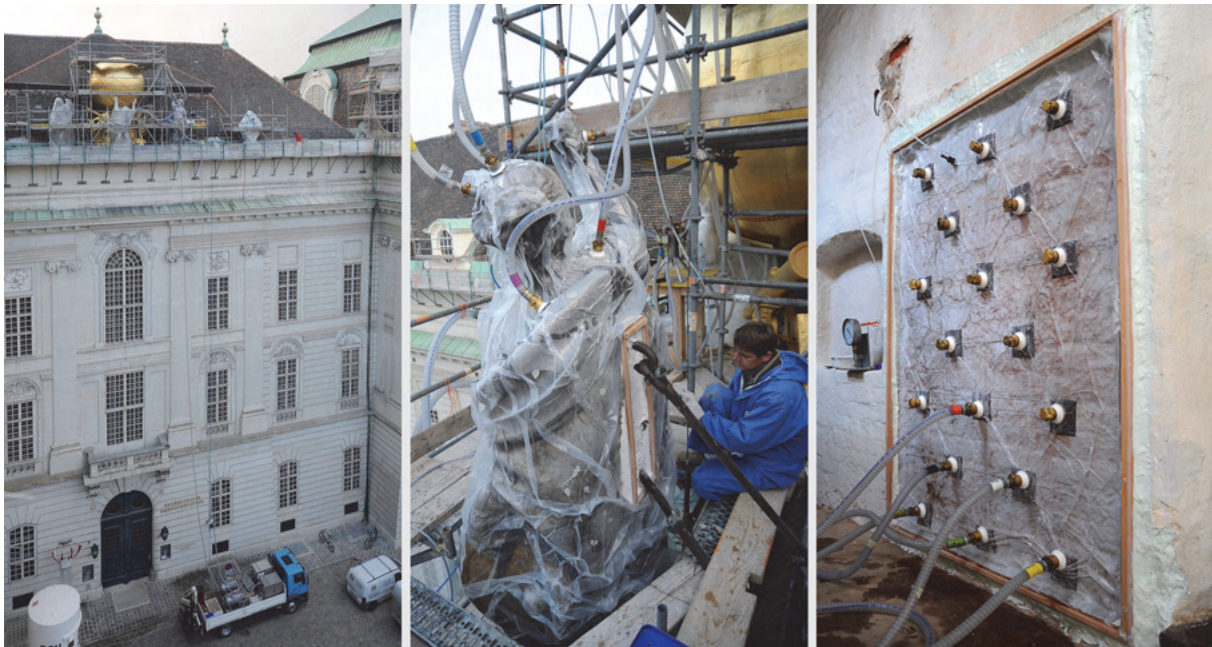
Fig. 2.1: First and second photograph: In-situ consolidation of 3-metre tall Attic sculptures of the National Library in Vienna which could not be dismantled. Two apparatuses (on the truck and at the sculpture) were coupled together to span the height of 30 m. Third photograph: Desalination of a brick wall over the full cross section. The wall was sealed on the front side to enable negative pressure on it. On the backside regular water was pressed into drilled injection valves. The desalination took six days of continuous flushing and about 2500 litres of water.
