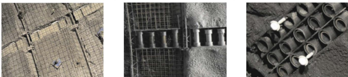
Fig. 7.6: Fotos of different types of lining segments (a) radial deformation, (b) tangential deformation (Mezger, F. et al. 2018)
