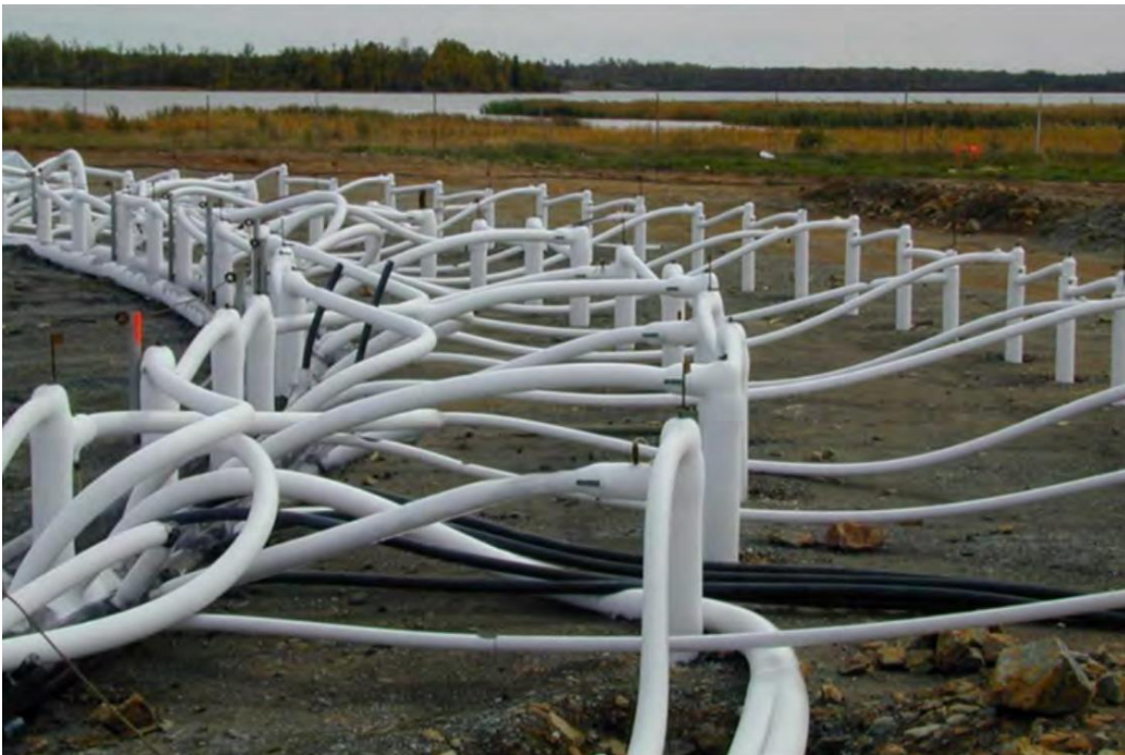
Fig. 4: Set-up of 3 rows of freeze pipes (Sopko & Auld, 2017)
