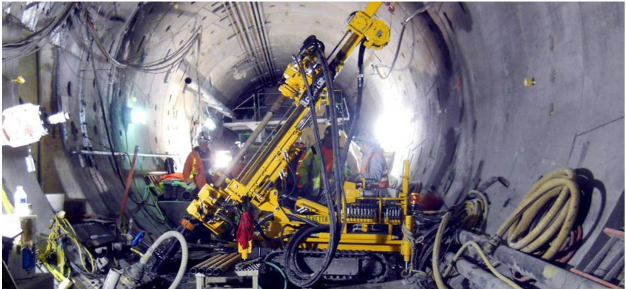
Fig 11: Permeation grouting in a tunnel (company material)
