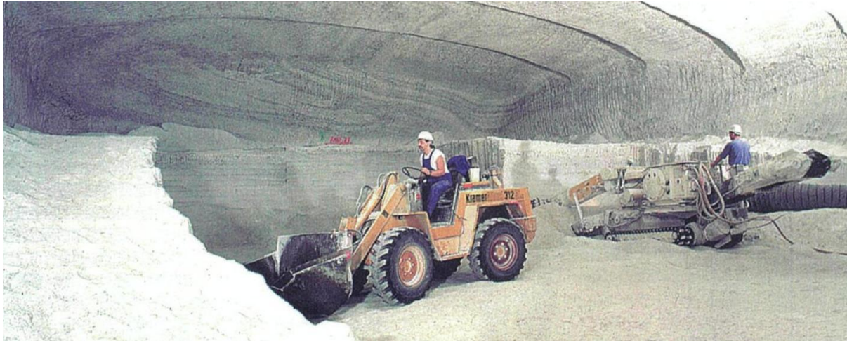
Fig. 8.12: Excavation process for concert hall in „Glückauf“ mine Sondershausen (Bartl, 2022)
