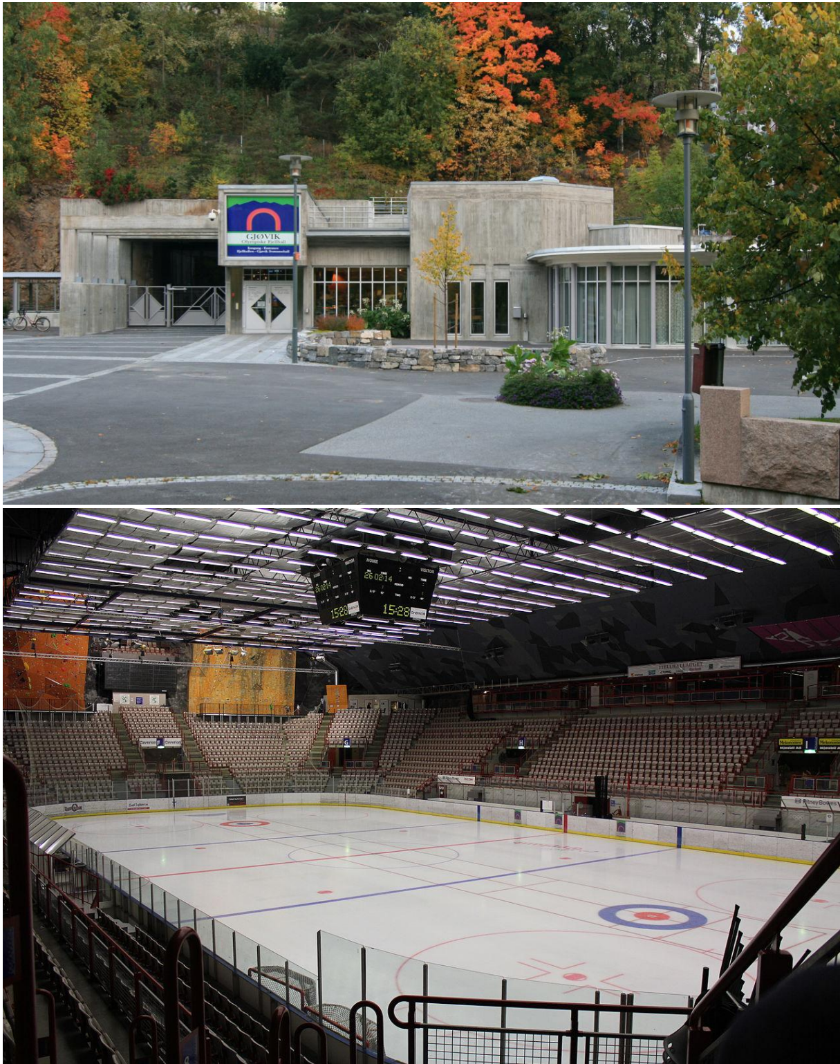
Fig. 8.3: Underground Gjøvik olympic cavern hall, Norway (Holmstad, 2014)
