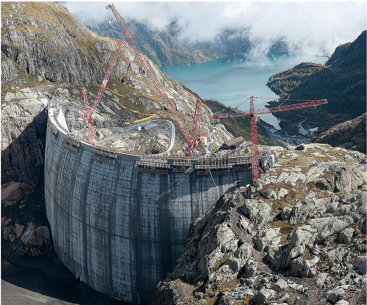
Fig. 2.16: Dam during construction (Nant de Drance HPS, company material)
