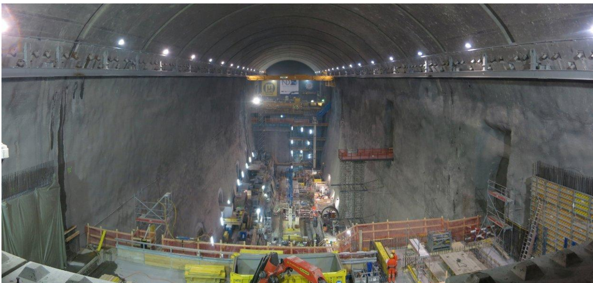
Fig. 2.14: Cavern during construction (Nant de Drance HPS, company material)
