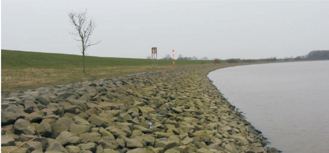
Fig. 9.7: Typical rip-rap revetment along a river bank (Mittelbach et al., 2014)
