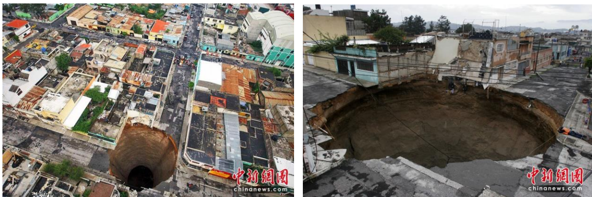
Fig. 11. Sinkhole (created by flooding and pipe leakage, Guatemala, 2010)
