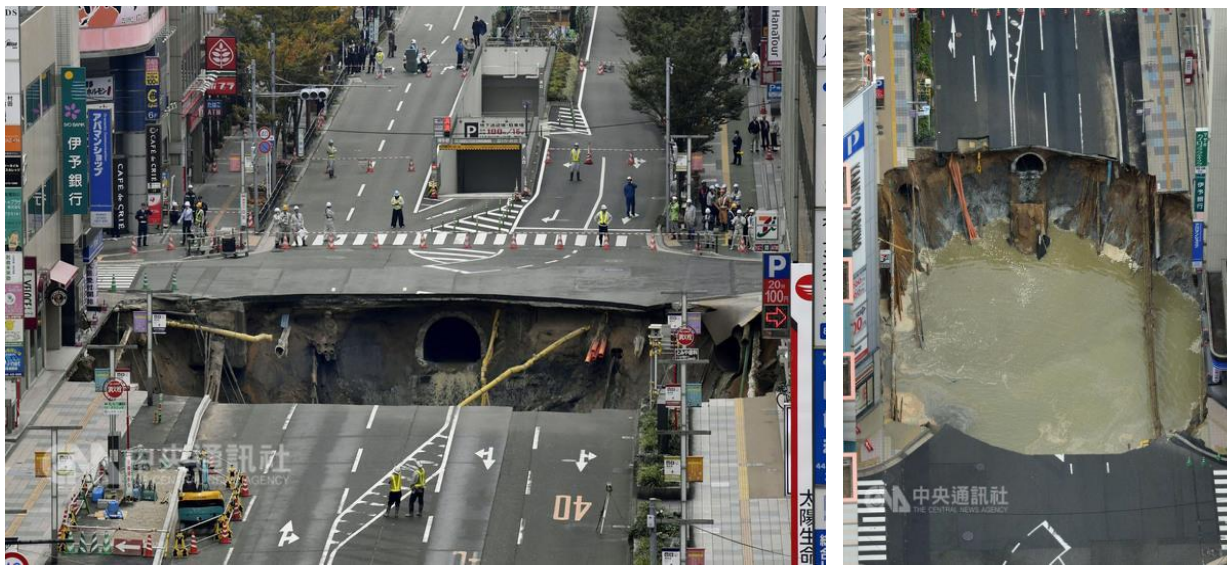
Fig. 10: Sinkhole (created by near surface tunneling, Japan, 2016)
