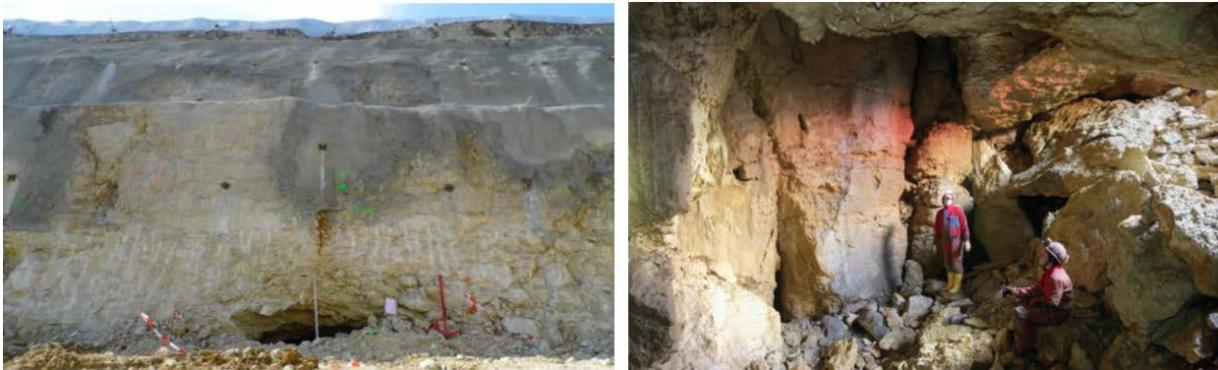
Fig. 4.8: Large karst cavities along the railway tunnel route Ulm-Wendlingen (Raithel et al., 2016)
