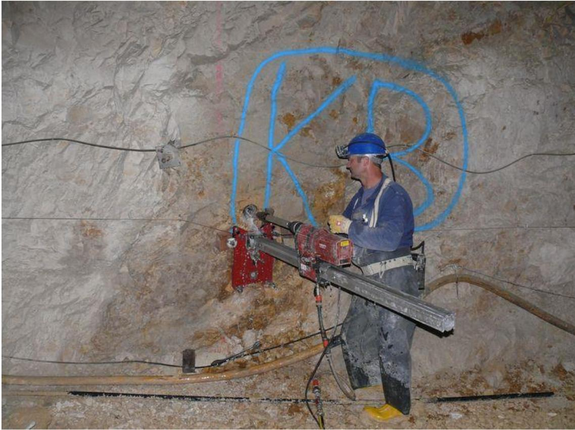
Fig. 21: Hammer-assisted hand drill with core drilling (RML 2016)
