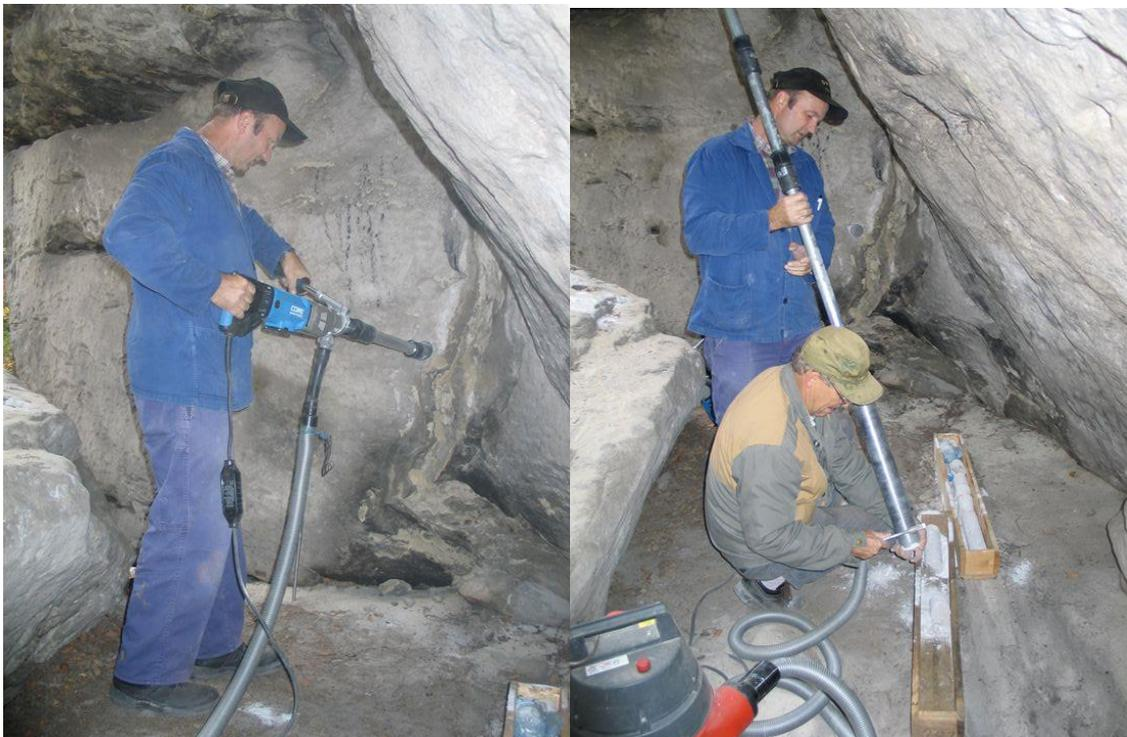
Fig. 22: Hammer-assisted hand drill with core drilling (RML 2016)
