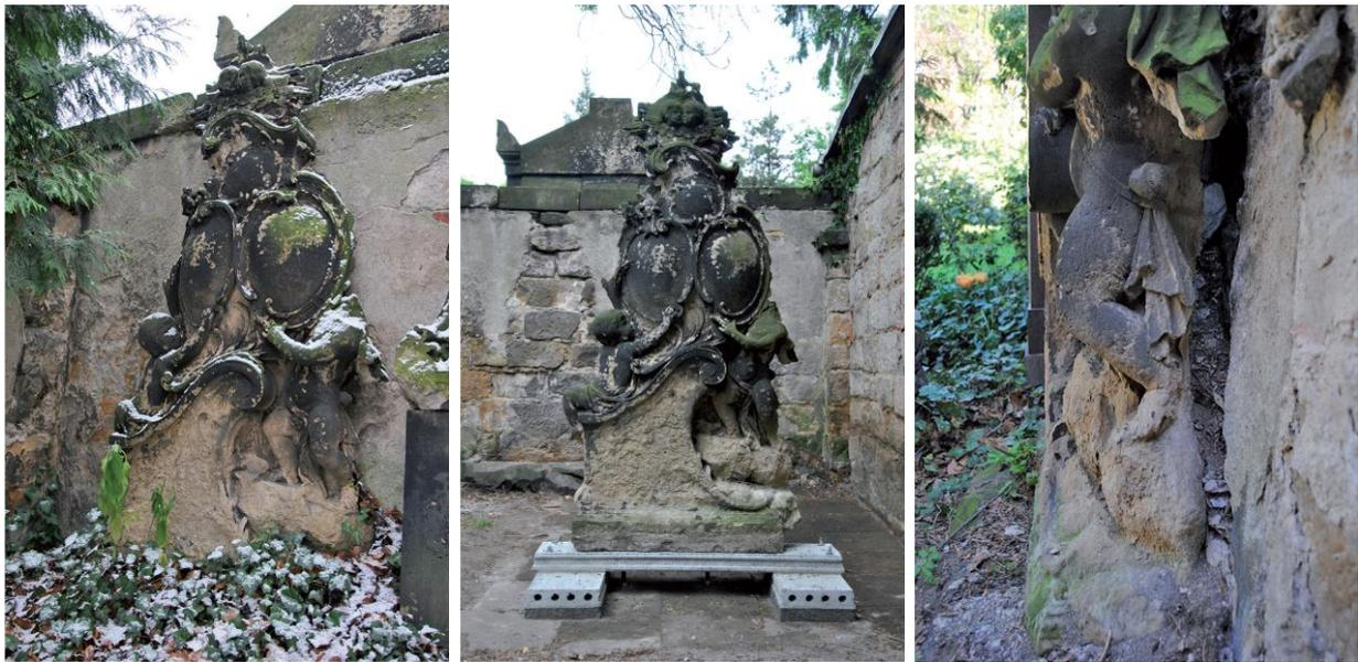
Fig. 2. Weathered baroque sandstone tombstone in Dresden [Wichert et al. 2018]
