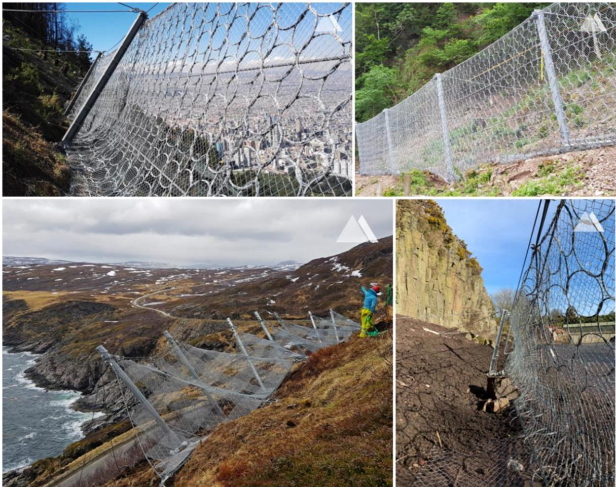
**Fig. 4.6:** Exemplary: flexible rockfall protection barriers in-situ (company material: Geobruigg)
