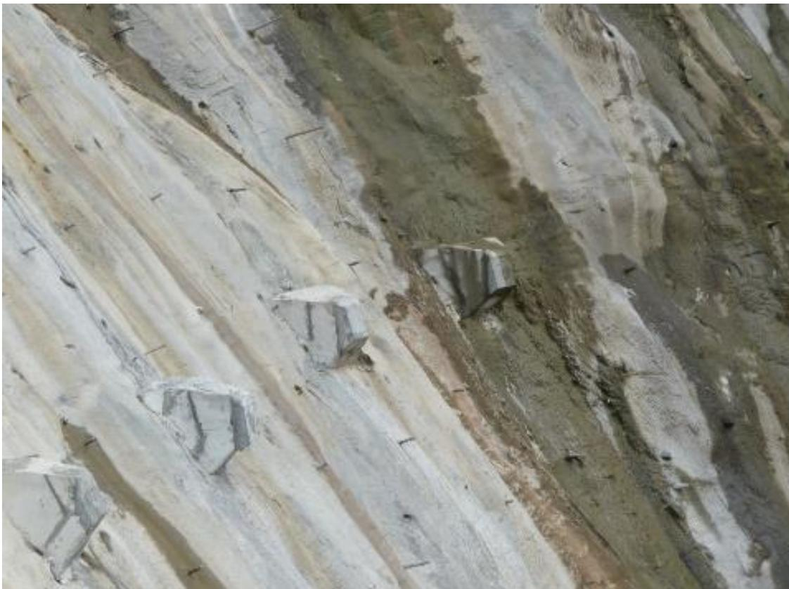
**Fig. 3.2:** Rock slope stabilised with berms, shotcrete, systematic pre-stressed anchorage and relief boreholes for dewatering (water dam project, China)
