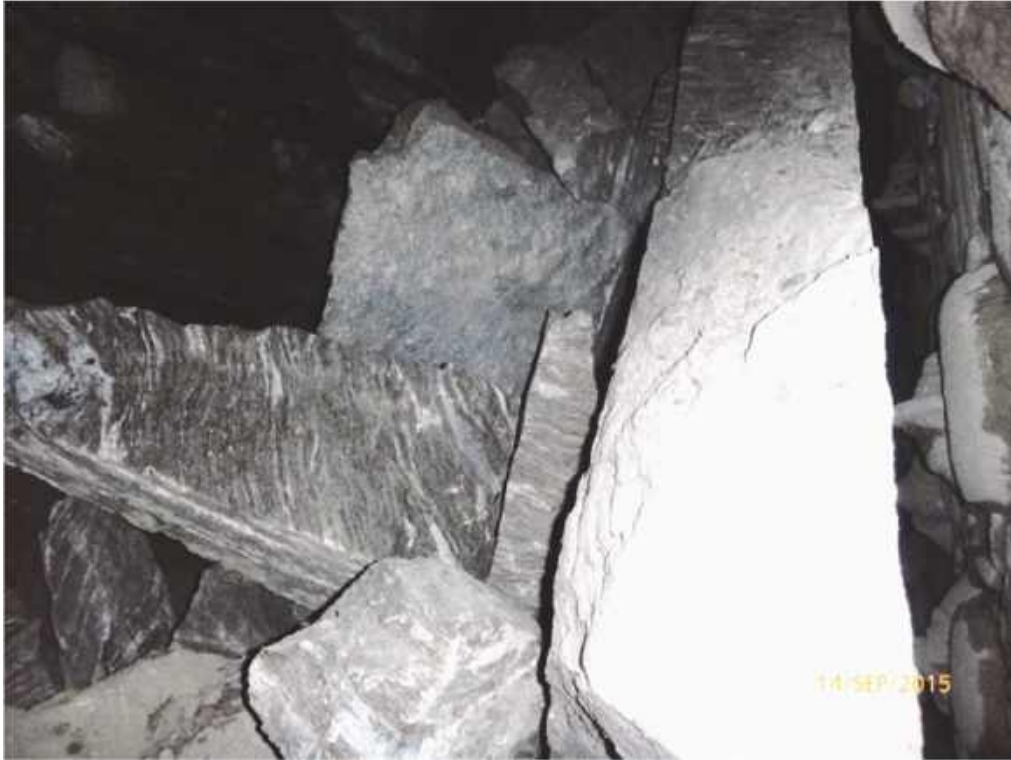
Fig. 3.5: Cubic decimetre to cubic meter large gneiss blocks in front of the cutterhead of a hard rock TBM. Discs and cutterhead can be seen on the right edge of the image (Photo: Plinninger).
