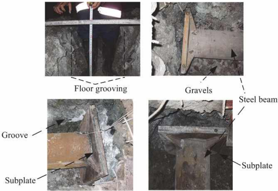
Fig. 16 The layout of floor beam in field experiment
