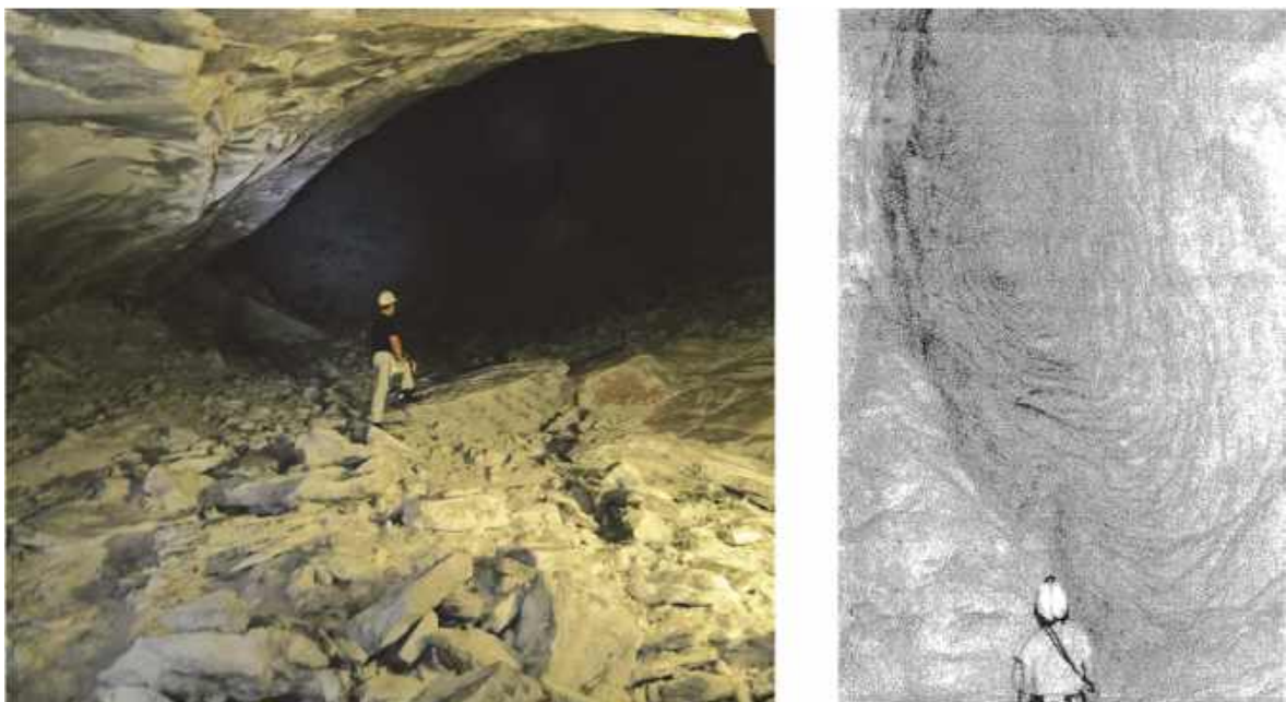
Figure 11: Outburst cavities. Left panel: Supercritical CO 2 in the Unterbreizbach mine (100 000 m 3 ), right panel: Hydrocarbon outburst in the Weeks Island salt dome (Davisson 2009).
