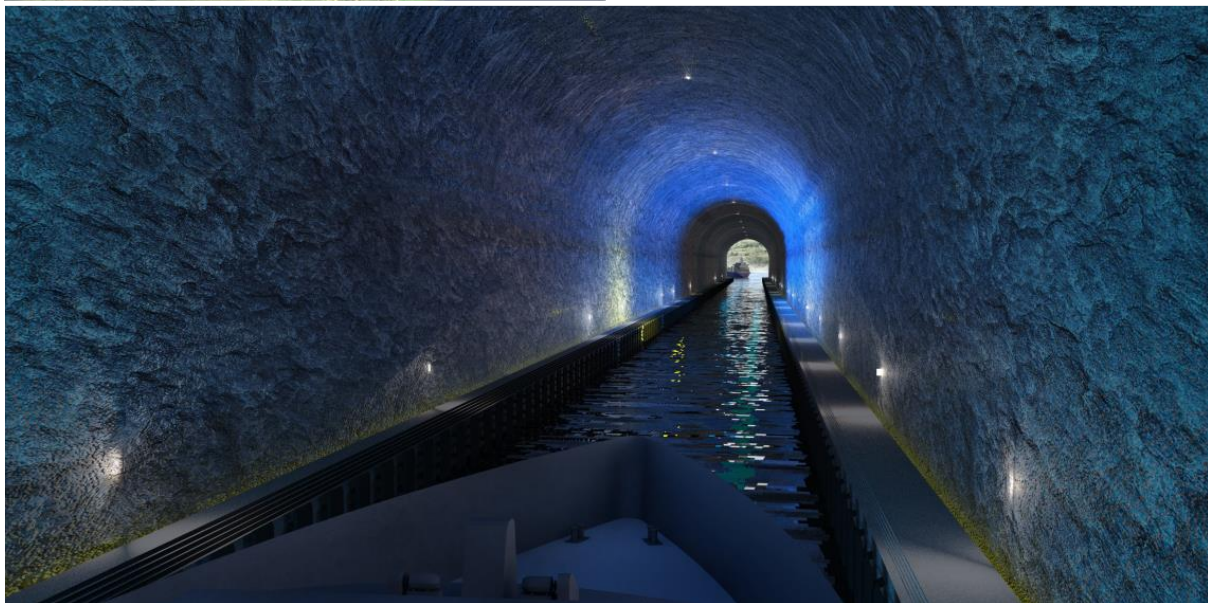
Fig. 5.3: Stad ship tunnel in Norway (Andreassen, 2018)
