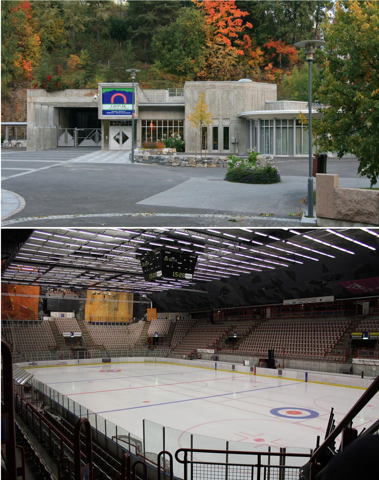
Fig. 8.3: Underground Gjøvik olympic cavern hall, Norway (Holmstad, 2014)
