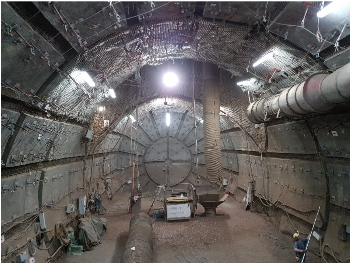
Fig. 4: Shotcrete shell with anchors and open compression slots.
