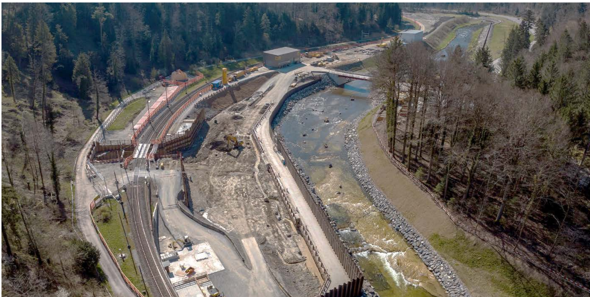
Fig. 6: The Sihl valley in spring 2023: cofferdam for building the intake structure; starting pit for TBM assembly, crossed by the provisional bridge for a local railway line; in the background to the right the existing driftwood rake at the outside bank [1].
