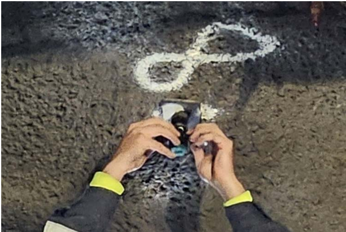
Fig. 20: The first prototype installation on-site.
