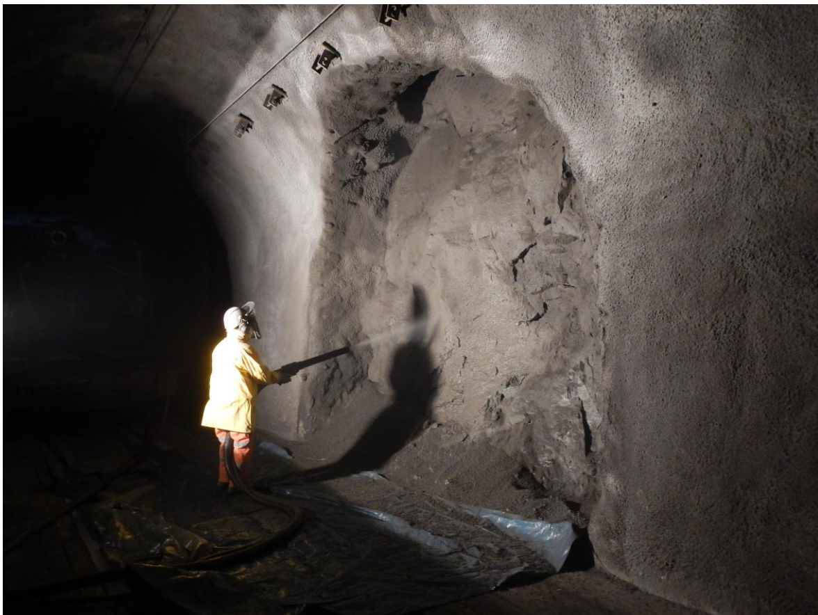
Fig. 6: Application of dry sprayed concrete (II) (Source:AF Toscana AG)
