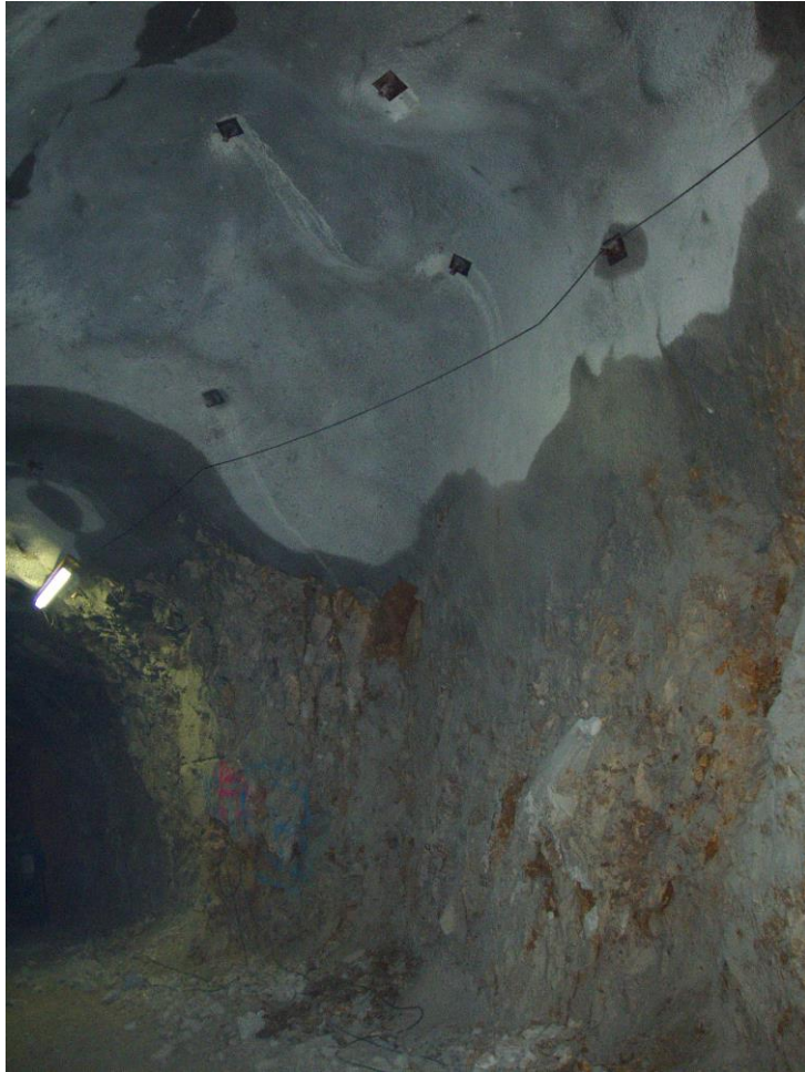
Fig. 1: Partial support with shotcrete in a mine
