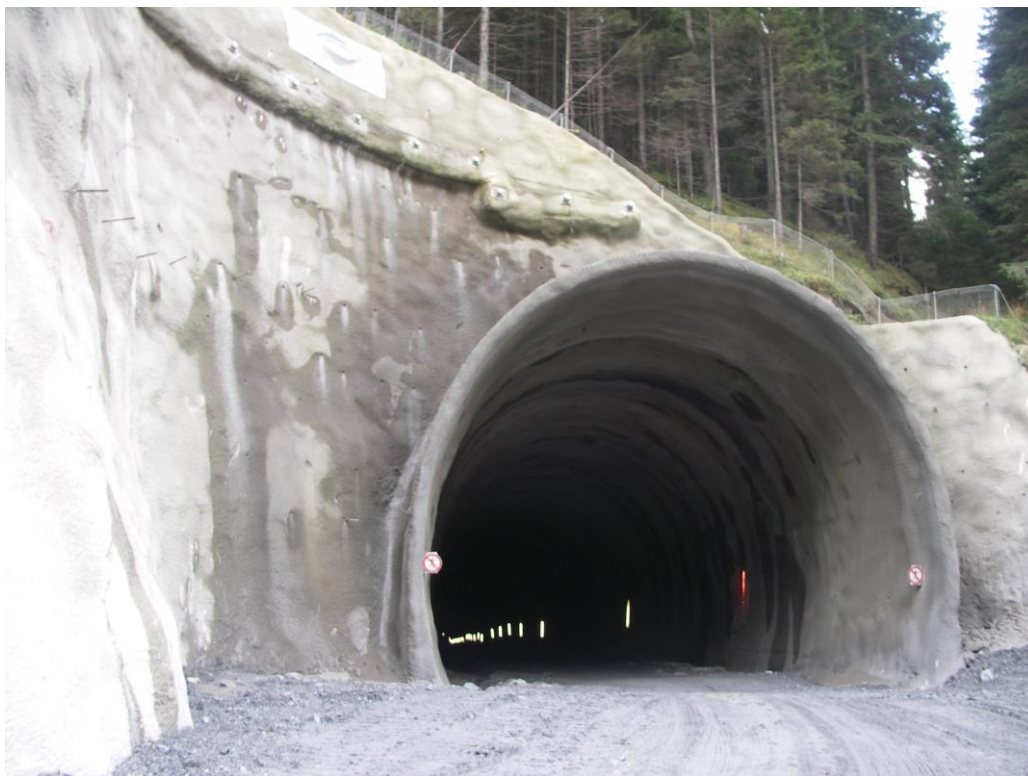
Fig. 2: Shotcrete application at a tunnel portal
