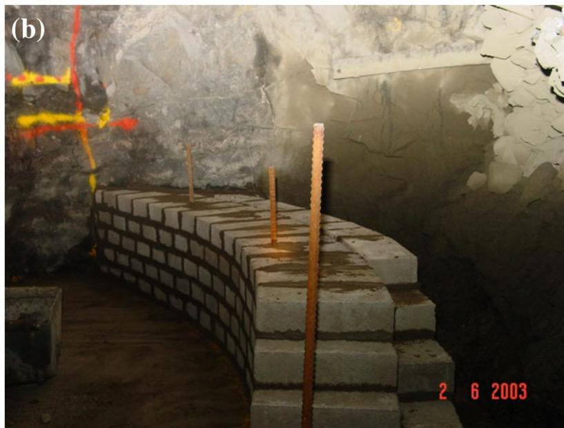
Fig. 2: Porous brick dam for hydraulic backfill (Sivakuga et al. 2015)
